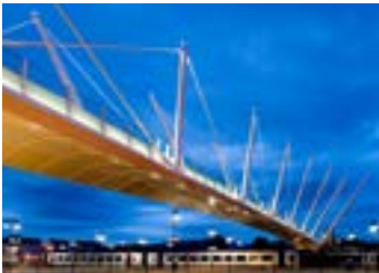
Forthside pedestrian footbridge
