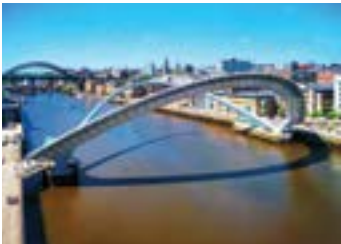
Gateshead millennium bridge
