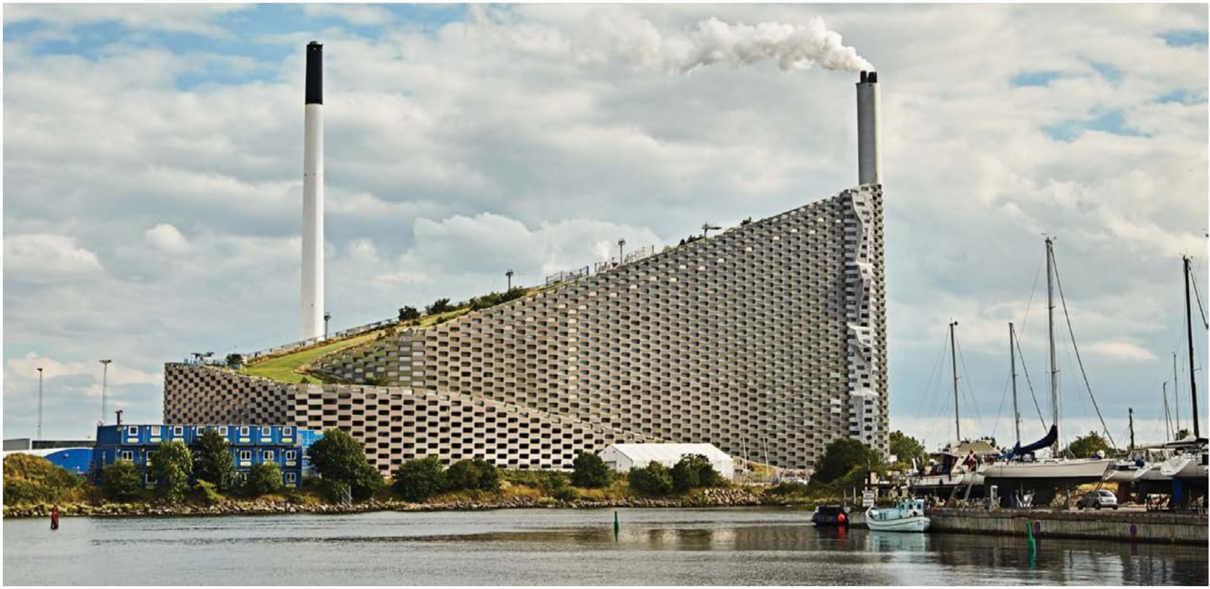
Copenhill is a combined heat and power waste-to-energy plant
