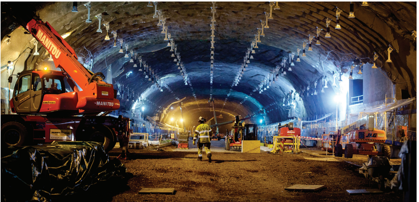
Image: Construction phase of Holmestrand Station
